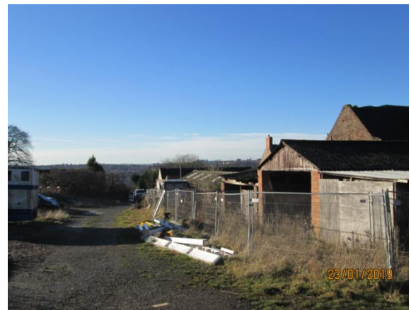
Barn to be House 4 including parts of building to be demolished.
