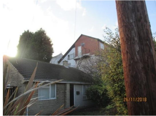
Rear of hotel (19 Meadow Road) in context with 2A
