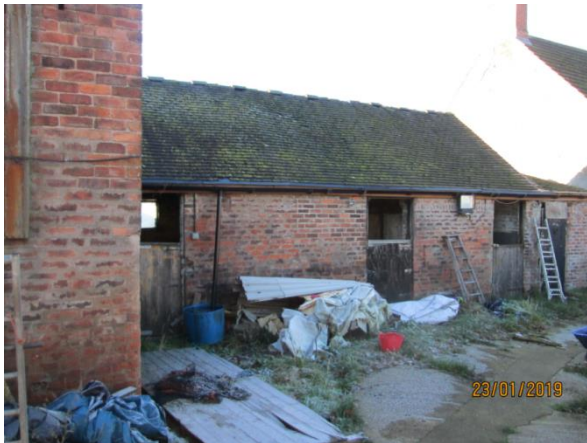
Rear elevation of barn to be House 5.
